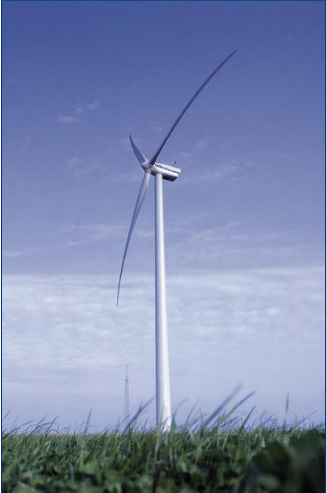
Figure 2.3: View of Wind Turbine
